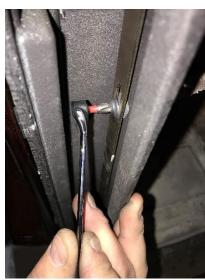
2) Install the new Push Rod. It is recommended to swap the Philips head screws removed in the previous step with the 10-24 Allen head screws provided in the kit. The Allen head screws are much easier to tighten properly in the confined space. Replacement washers and bushings are also provided should replacement hardware be necessary. See picture for proper assembly order.
